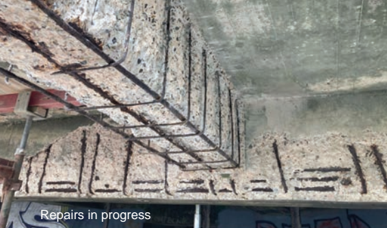
Repairs in progress
